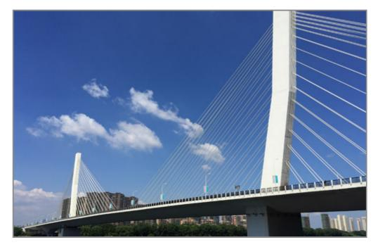
Completed in December 2003, Fumin Bridge is a 602 m (2,000-feet) long cable-stayed bridge over the Hun River in Shenyang, China. At a height of 67.5 m (223-feet) and 32.5 m (107-feet) wide, it accommodates two lanes of traffic in each direction. It connects Shenyang's Fengle district with Hunan District on the southern riverbank.
