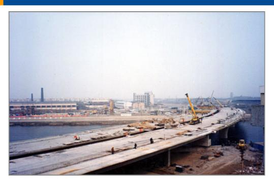
Located in Tianjin, China, the HaiHe River Bridge connects the city's Hedong District with the Jianshan District on the southern riverbank. The HaiHe River Bridge has a length of 868 m (2,870-feet) and a width of 39.5 m (130-feet) to accommodate a two-way, three lane highway. The three-span continuous beam design employs intermediate shaped concrete piers as foundations.
