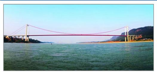
Nanxi Bridge was opened in 2012 as part of the G93 Chengdu-Chongqing Ring Expressway across the Yangtze River in Nanxi District, Yibin, Sichuan in China. With a span of 820 m (2,700-feet) and a total length of 1,295 m (4,300-feet), the Nanxi Bridge is one of the longest suspension bridges in the world. The USD 95-million project is 24.5 m (81-feet) wide and accommodates a two-way four-lane highway designed for speeds of up to 80km/h (50-mph).
