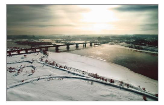
Irkutsk, Siberia's largest city, is bisected by the Angara River. As a key part of the city's transport infrastructure, the Irkutsk Bridge is 1,625 m (5,360-feet) long and 32 m (106-feet) wide. Construction work on the bridge was conducted in harsh climatic conditions; in-situ pre-stressed reinforced concrete was used.
