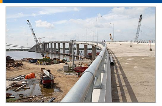
My Loi Bridge is located in the Mekong Delta province of Tien Giang. The bridge opened to traffic on August 2015. It is 1,422 m (4,700-feet) long and 12 m (40-feet) wide and was completed after only 18 months of construction. My Loi Bridge helped reshape the transport route in the Southern region by spanning the Vam Co River and replacing a ferry service, reducing the travel distance from Go Cong to Ho Chi Minh City from 100 km (62 miles) to 25 km (16 miles).
