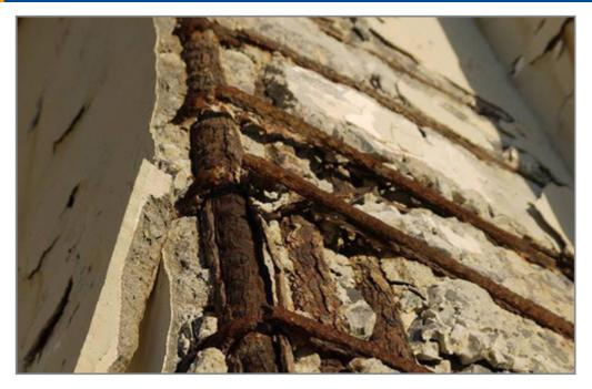
A worldwide challenge, corrosion of reinforcement steel is the main reason for concrete deterioration. Failure of concrete structures due to corrosion has major safety implications for critical infrastructure, such as highways, tunnels, bridges and other projects exposed to aggressive environments. The National Association of Corrosion Engineers (NACE) in the USA estimates the direct cost of corrosion for highway bridges alone to be USD 13.6 billion *every year*.
