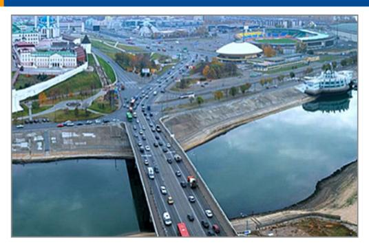
While the new, eight-lane bridge over the Kama River inherited the previous Soviet name, it was totally rebuilt after more than 50 years of service. The new bridge features eight lanes and a separate pedestrian zone. The total length of the bridge is 172 m (570-feet).
