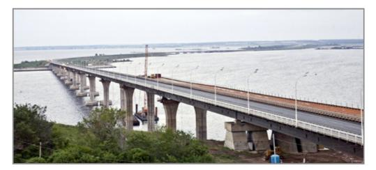
The Kama Bridge is a part of the longest artificial road structure in Russia (as measured by the length of elevated roadway). With a total length of 14 km (9-miles), the structure has three bridges: over the Kama River (1,608 m / 1-mile), over the Arkharovka River (550 m / 1,815-feet) and over the Kurlyanka River (70 m / 230-feet). The bridges are a key part of the major Kazan-Chistopol-Bugulma-Orenburg Highway.
